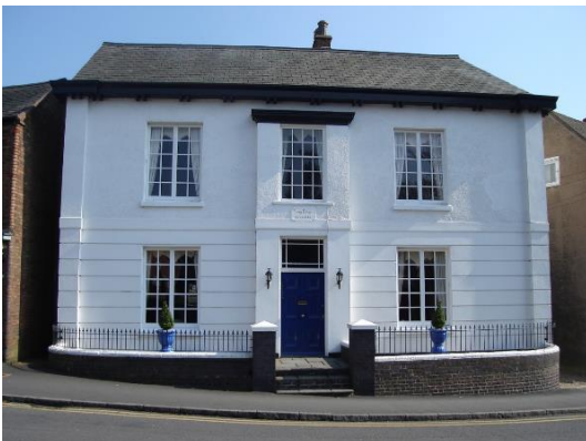
Tong Lodge, Church Street
